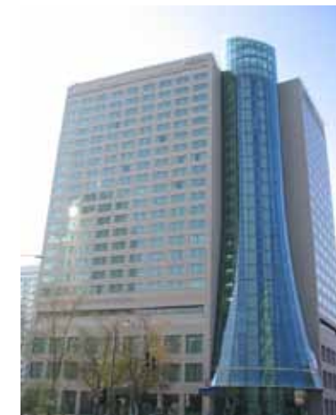
The Westin hotel in Warsaw invested in a security solution consisting of mechanical and electromechanical lock cases, a Master Key System, card readers and panic exit devices.
