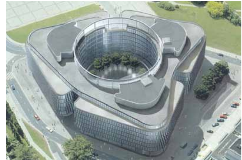
The Metropolitan is an office center in Warsaw, designed by Norman Foster. ASSA has over 2.500 cylinders in a Master Key System installed within the building.
